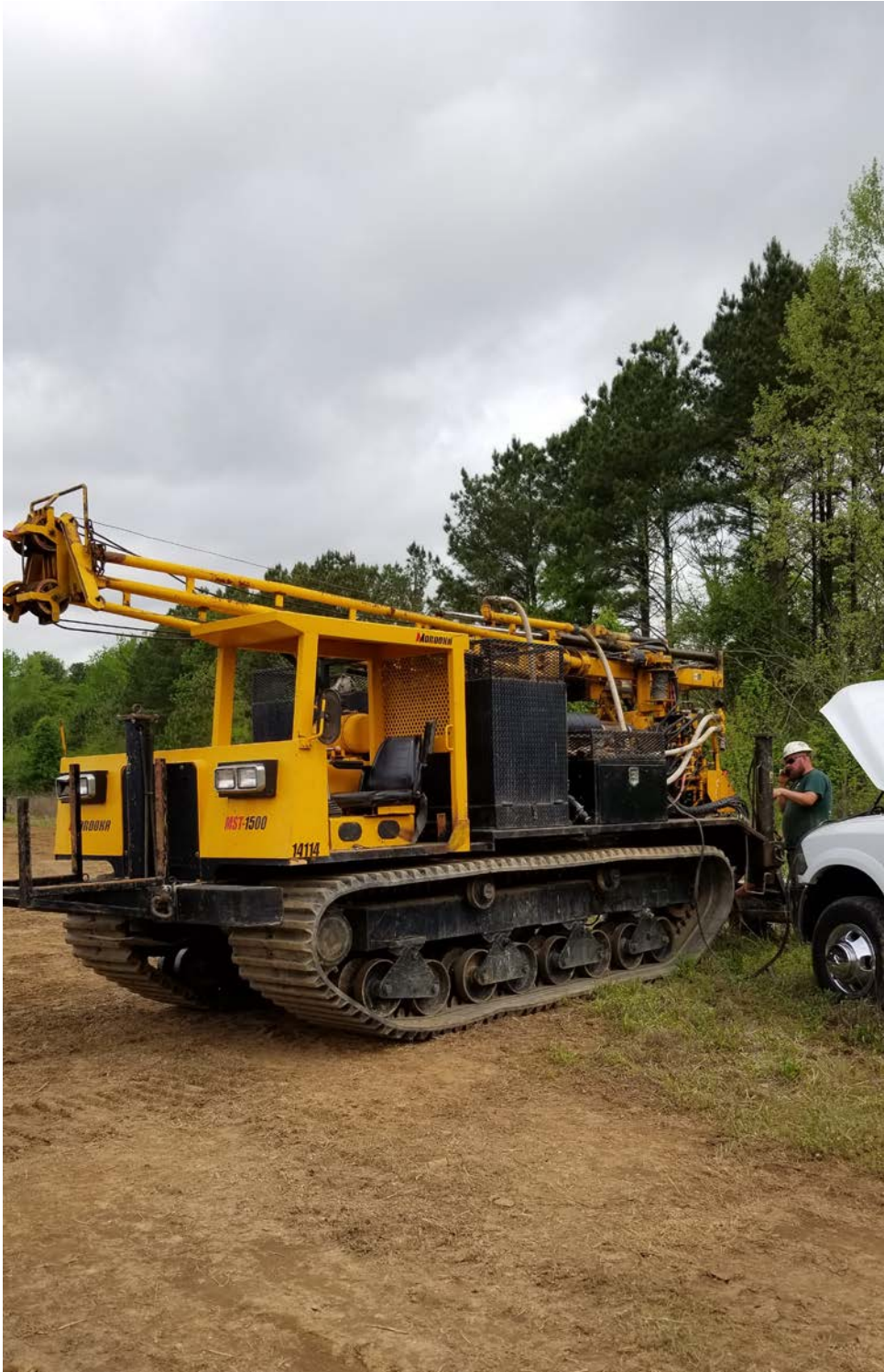
Figure 1: SPT drill rig.
