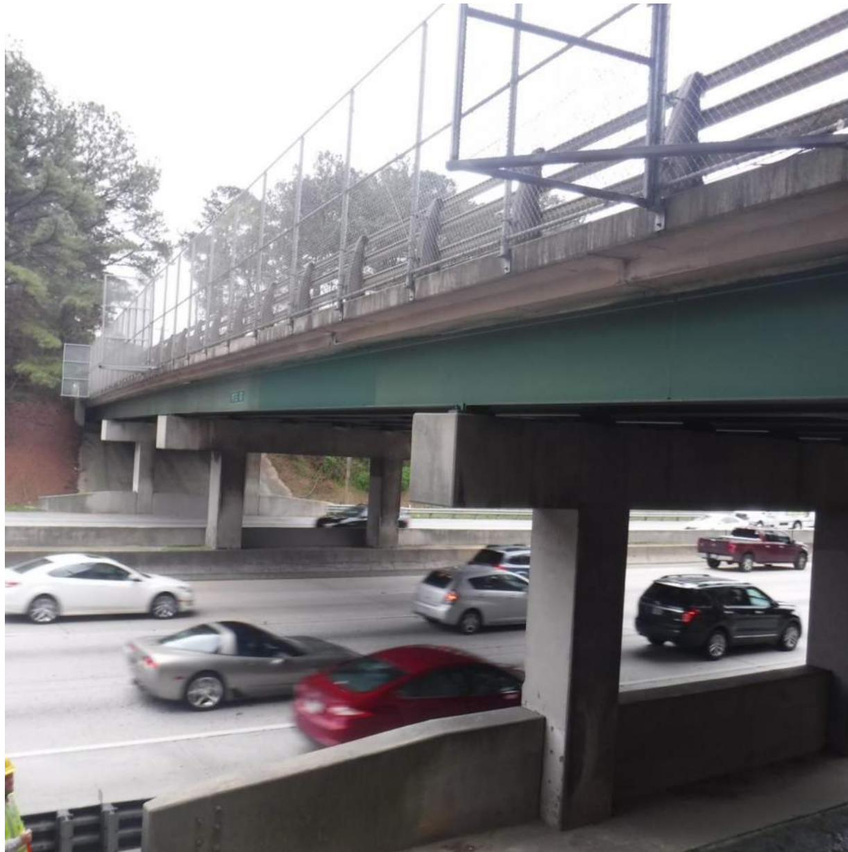
FIGURE 1 Pitts Road over SR 400 EXISTING BRIDGE
